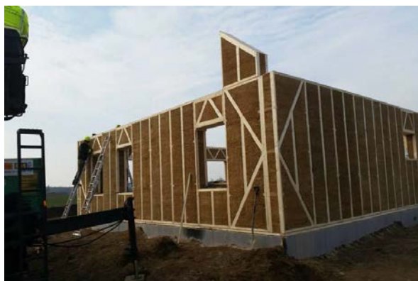
Fig. 2. Frame system with straw panels
